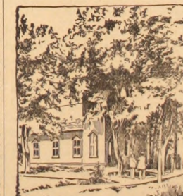
PRESENT CLUB HOUSE, Old Presbyterian Church.
