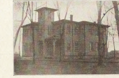
EAST SIDE SCHOOL BUILDING.
