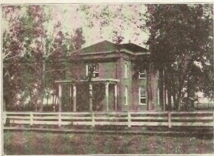
WEST SIDE SCHOOL BUILDING.
