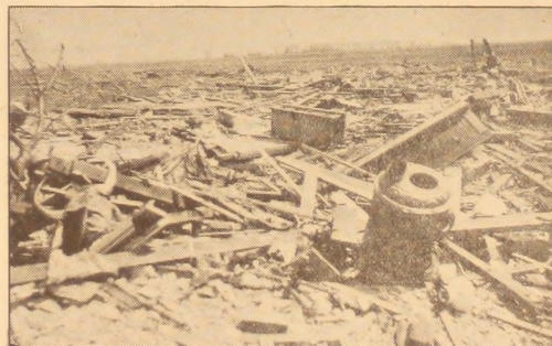
Site of the farm of L. P. Reimer on the Kern farm, two miles south and one-half mile west of here, which was completely demolished, leaving buildings and household goods scattered across the field.
