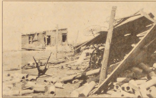
A picture of the Sorensen farm where Andrew Anderson lives. All of the buildings being partially destroyed, leaving a mass of ruins on the farm.
