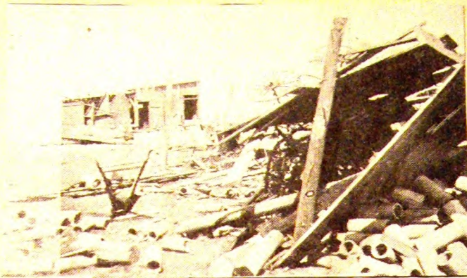
RUINS ON THE KERN FARM FOLLOWING THE TORNADO OF APRIL 21, 1912
