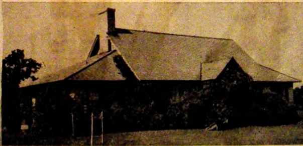
Formally opened to the membership on September 22, 1924. The building is situated on a knoll near the creek and faces the north. There is a large main room which has a fireplace on the east side. Along the entire south side is an enclosed porch which opens from the main room. The Dwight Country Club was organized approximately twenty-five years ago, and from a small organization has grown to a large substantial membership. The attractive grounds afford many pleasant hours for the devotees of golf, during the summer months, and many social activities have taken place at the club house during past years, well as tournaments, both local and inter-city, on the golf grounds. Hans P. Rosendall is the President this year of the Club.
